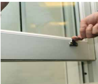
Optional Deep bottom rail with traditional jointing
